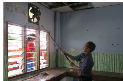
Shafiee from Human Resource Department removing the peeled paint before putting up a fresh coat
